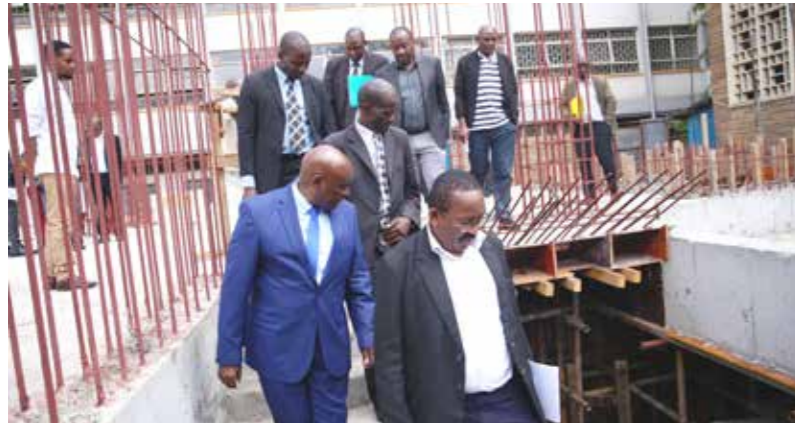
The VC, Prof Benedict Mutua tours the construction site of I-Block
